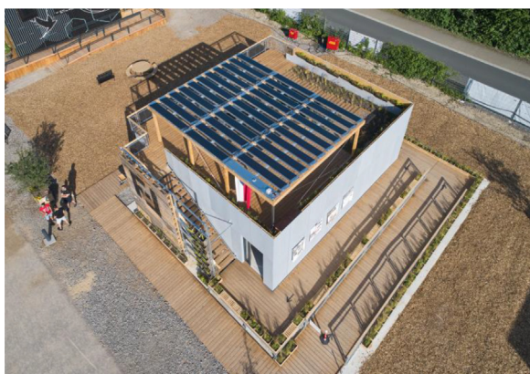
Fig. 19. Non-visible thin film PV on the saw-type metal roofing of the CTU house © Sigurd Steinprinz, University of Wuppertal.
