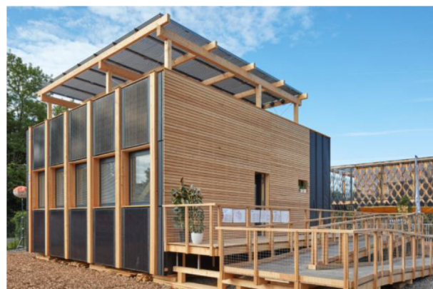
Fig. 20. Black, vertical PVT collectors on the east façade, and horizontal thin film PV tubes covering the roof garden of the HBC building © Sigurd Steinprinz, University of Wuppertal.
