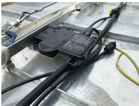
Fig. 23. Rear side of a 250 W PVT module with integrated inverter (GRE).
