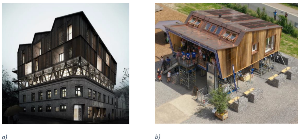
Fig. 2. The overall winner, Team “RoofKIT”. Illustration of the design challenge contribution with a vertical extension of an existing building in Wuppertal (a) and photo the representative demonstration unit on the competition site (b). Illustration: Team RoofKIT, Karlsruhe Institute of Technology, Photo: SDE 21/22.
