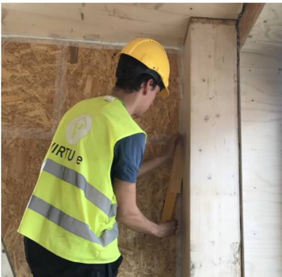
Fig. 7. A student from the TUE Team masking the joints of prefabricated façade elements for air tightness.
