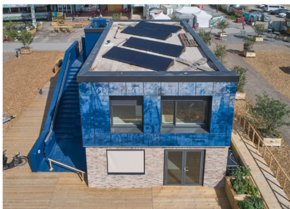
Fig. 18. Roof mounted, non-visible standard PV modules together with blue ceramic image print PV on the south façade of the TUD house © Sigurd Steinprinz, University of Wuppertal.
