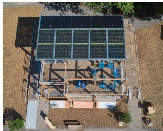
Fig. 21. Daylighting PV modules (front) and PVT collectors (back) cover the roof terrace of the GRE house © Sigurd Steinprinz, University of Wuppertal.
